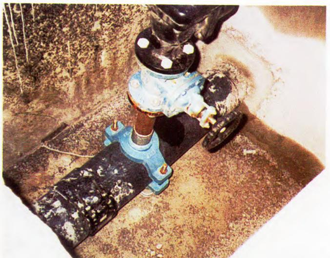
200 mm  $\varnothing$  HDPE pipe connected with air valve in Oman
