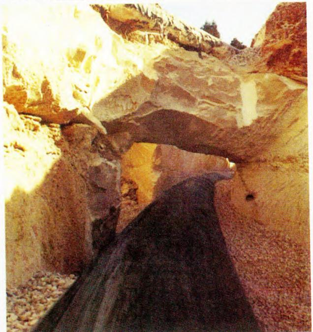
16" SDR 11 pipe passing under a high pressure natural gas line.
