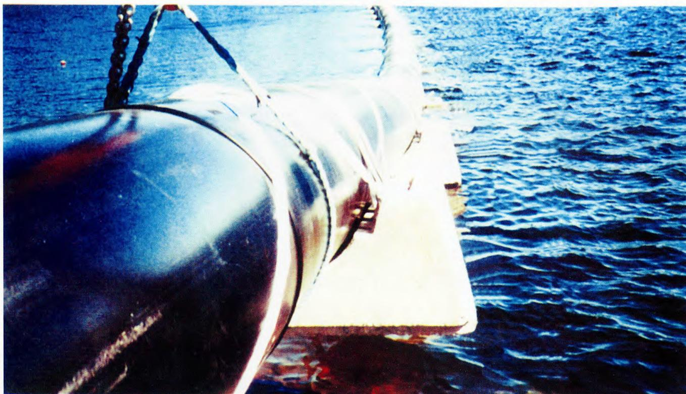
**H**igh Density Polyethylene (PE-HD) pipes have been used for more than forty years. The experience shows evidence that PE-HD pipes offer an optimal solution to most pipe problems. PE-HD pipes have outstanding advantages over conventional materials, such as:
