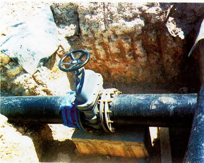
315 mm  $\varnothing$  Sewage line connected with gate valve in Oman
