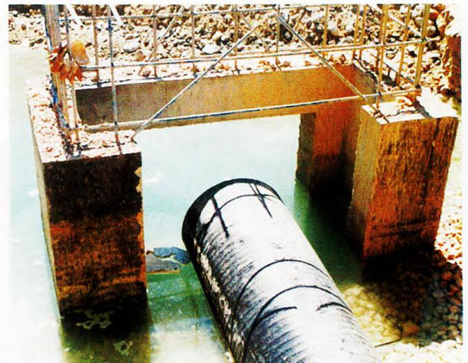
600 mm to 1200 mm  $\varnothing$  HDPF Weholite pipes for storm water drainage at port, in Oman.
