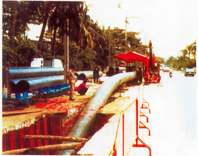
Relining of old leaking water pipeline in Bangkok, Thailand. Dimensions  $\varnothing$  355 - 710 mm. Total length 9 300 mm.
