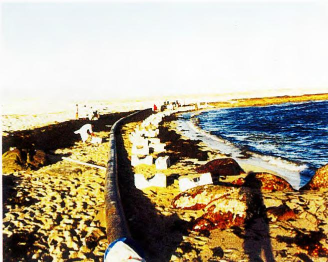
315 mm  $\varnothing$  seawater intake pipeline in Oman.
