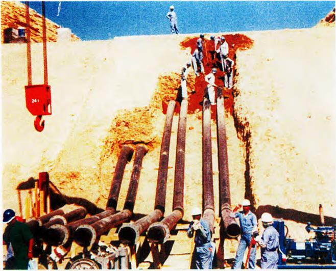
315 mm to 500 mm  $\varnothing$  drainage facility in Oman.
