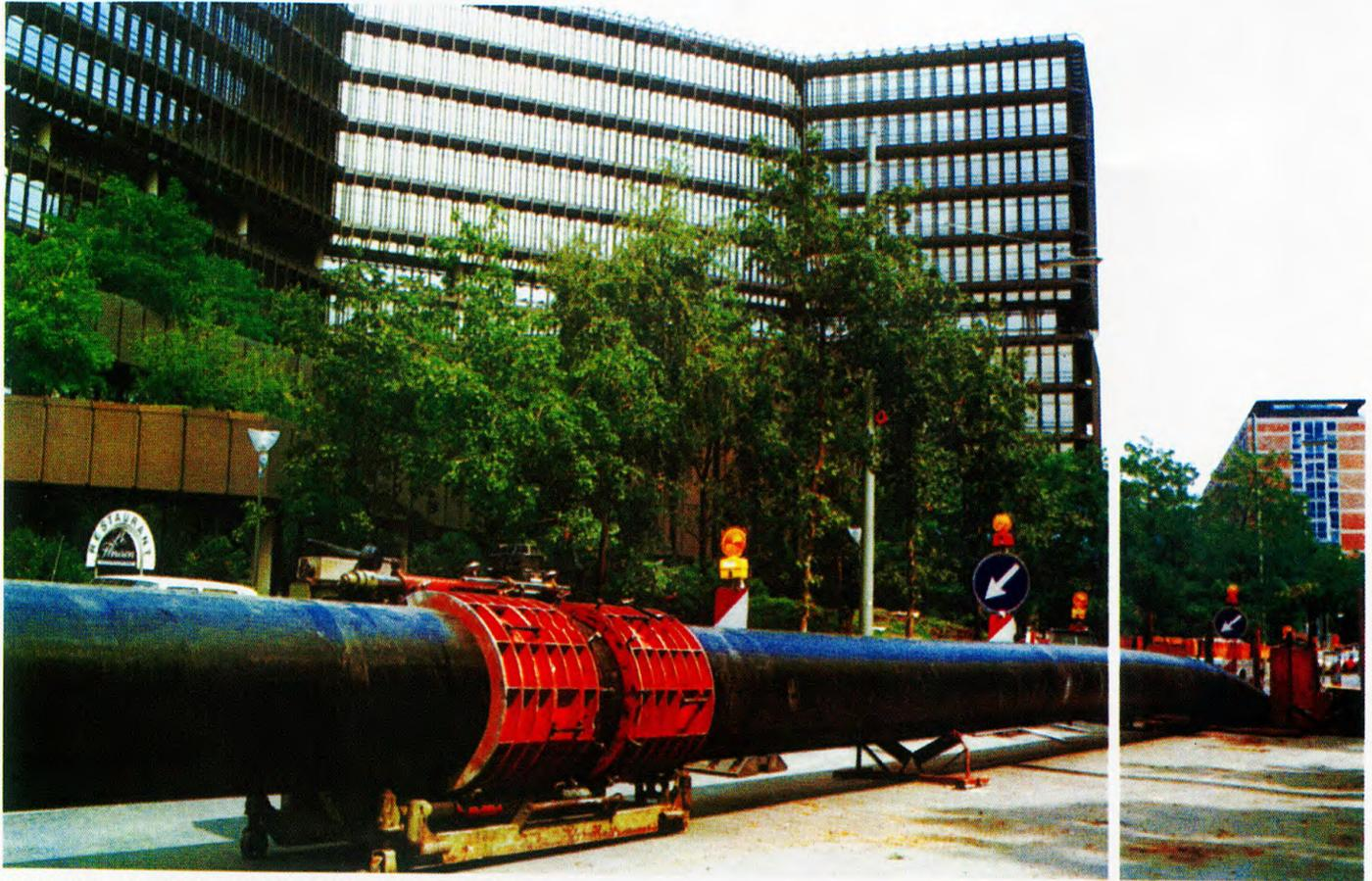
*Installation of ø 900 mm PE-HD pipe in Munich, Germany*
