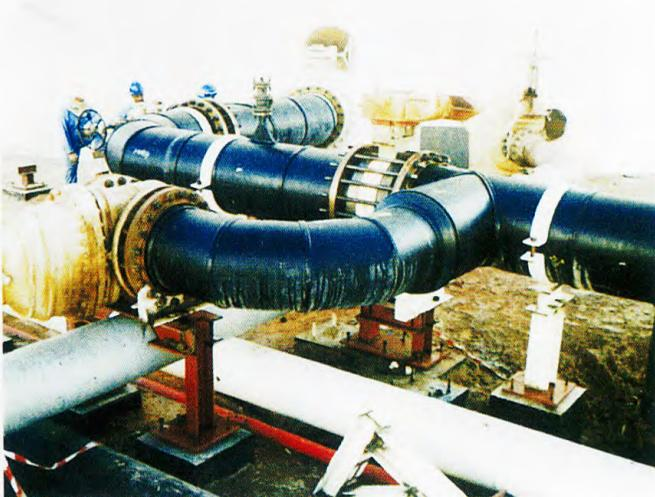
Replacement of Carbon Steel pipes with HDPE for crude oil with all interconnections, in Oman.
